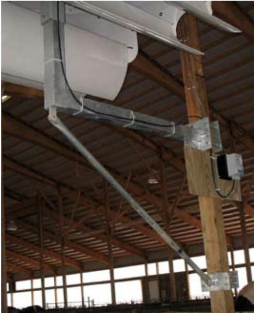
Figure 7 - Absolute Air install on a column
